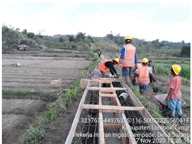
4 Construction work progress 50%
