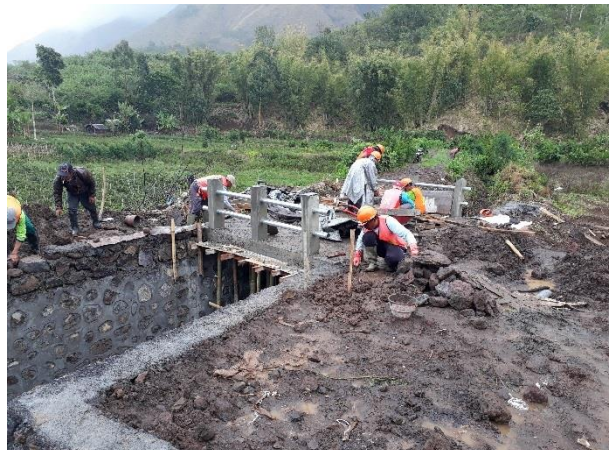
4 Construction work progress 50%
