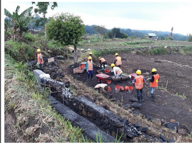
3 Construction work progress 25%
