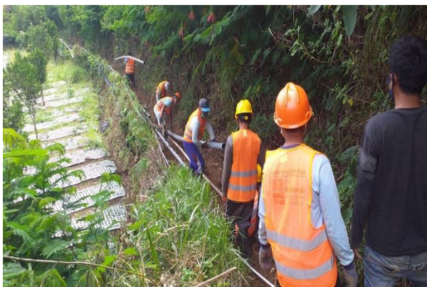
3 Construction work progress 25%
