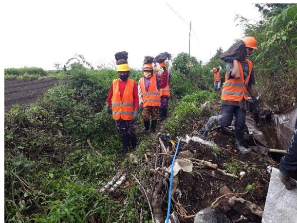
2 Preparation work i.e. material mobilization
