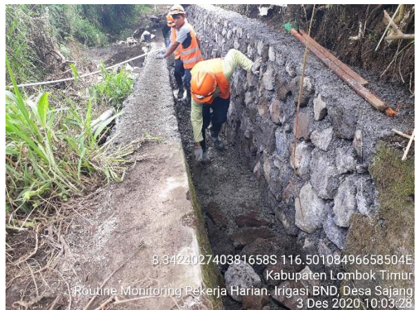
4 Construction work progress 50%
