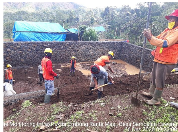
4 Construction work progress 50%
