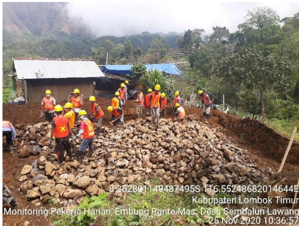
3 Construction work progress 5%
