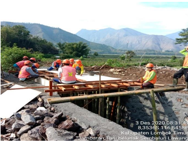
3 Construction work progress 25%
