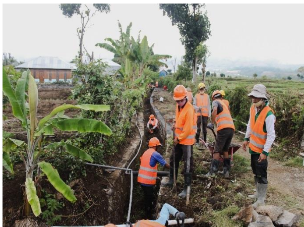
3 Construction work progress 25%
