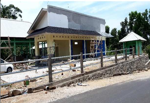
5 Construction work progress 75%
